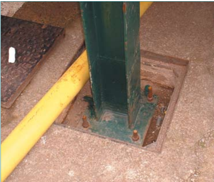
Figure 5 Permanent base for regular re-use
