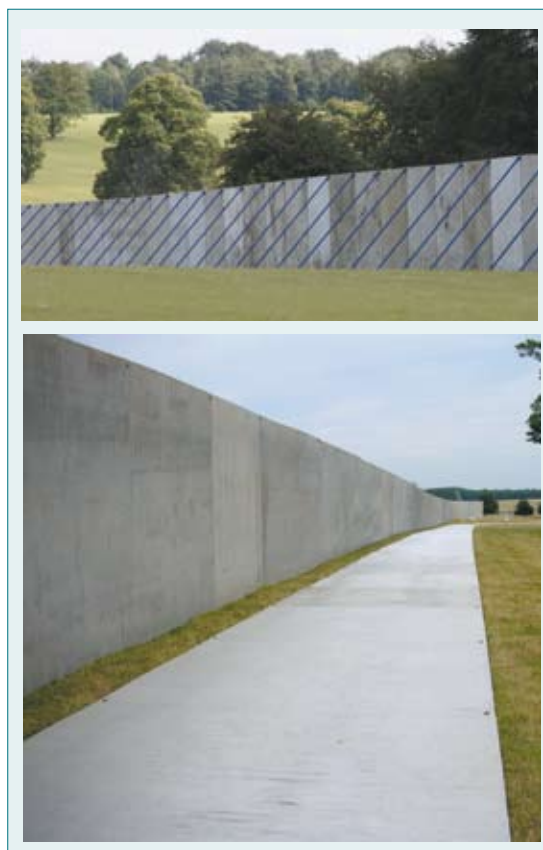
Figure 34 Roadway panel fencing
