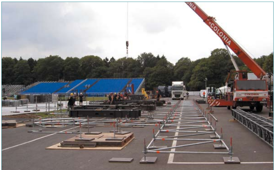
Figure 2 A site in part-built mode
