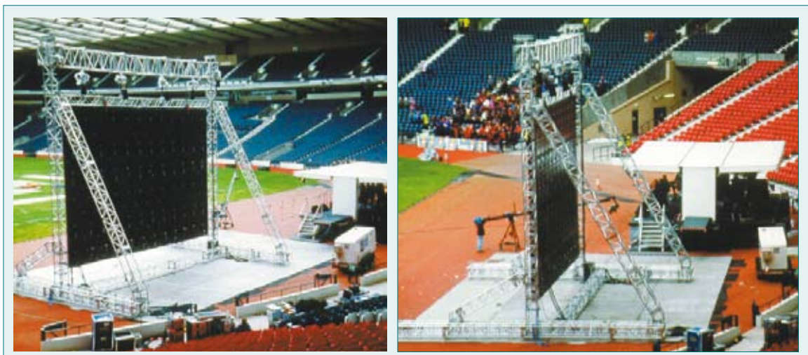
Figure 45 Video screen support structure
