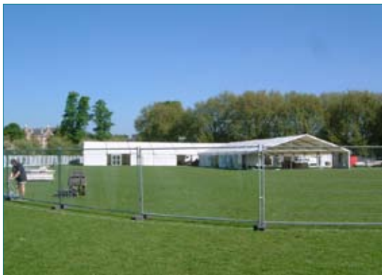
Figure 31 Mesh Panel fencing
