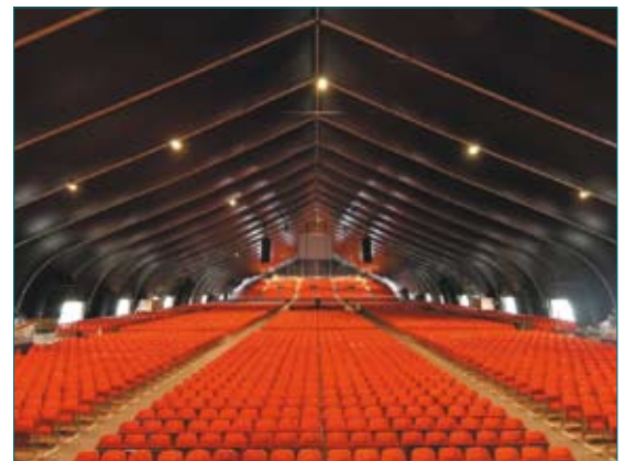
Figure 43 The interior of a large framed marquee
