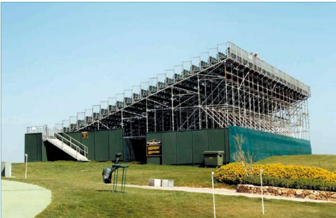
Figure 14 Temporary grandstand erected for a golf tournament
