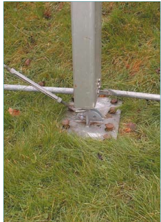
Figure 6 Frame marquee base plate
