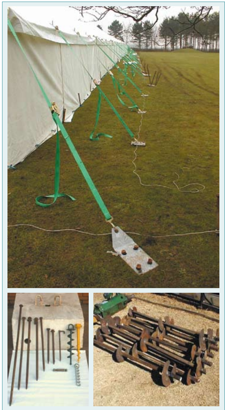
Figure 7 Ground anchors
