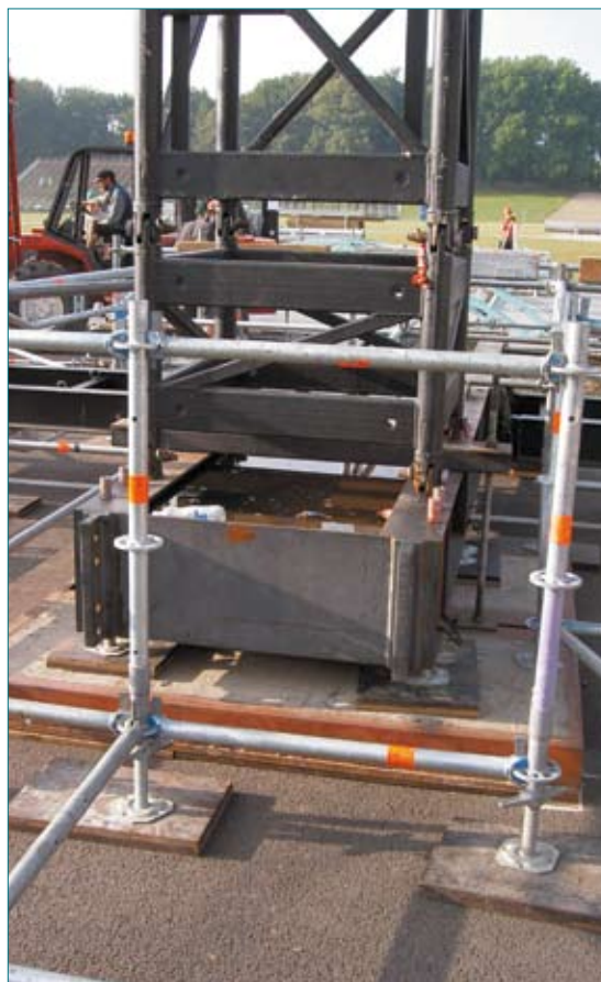
Figure 10 A heavy duty substructure arrangement
